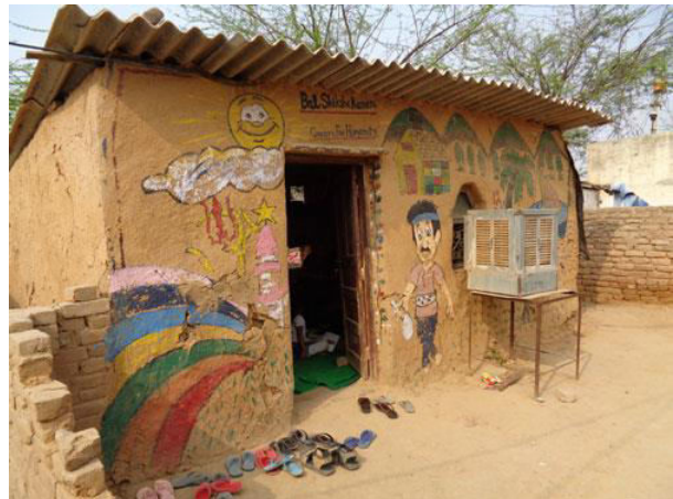
Learning Centre with a small fenced yard.
